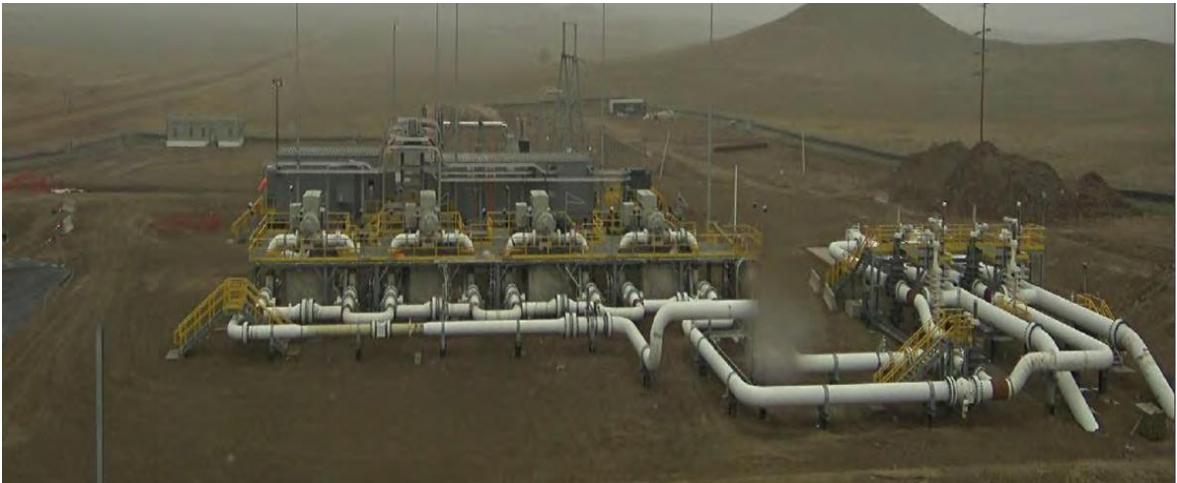
PUMP STATION 14 – 12 th April 2021
