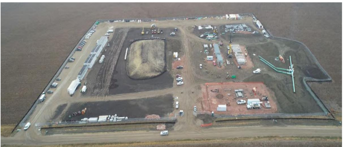
PUMP STATION 18 – October 2020
